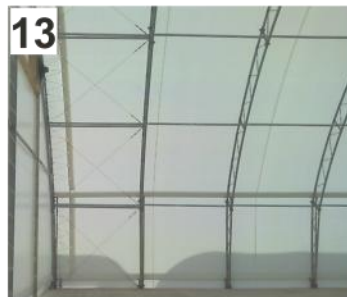
65 and 72 Building Leg Bracing
